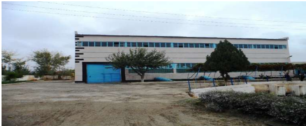
Figure 1.1. Main building of the pumping station” satellite
