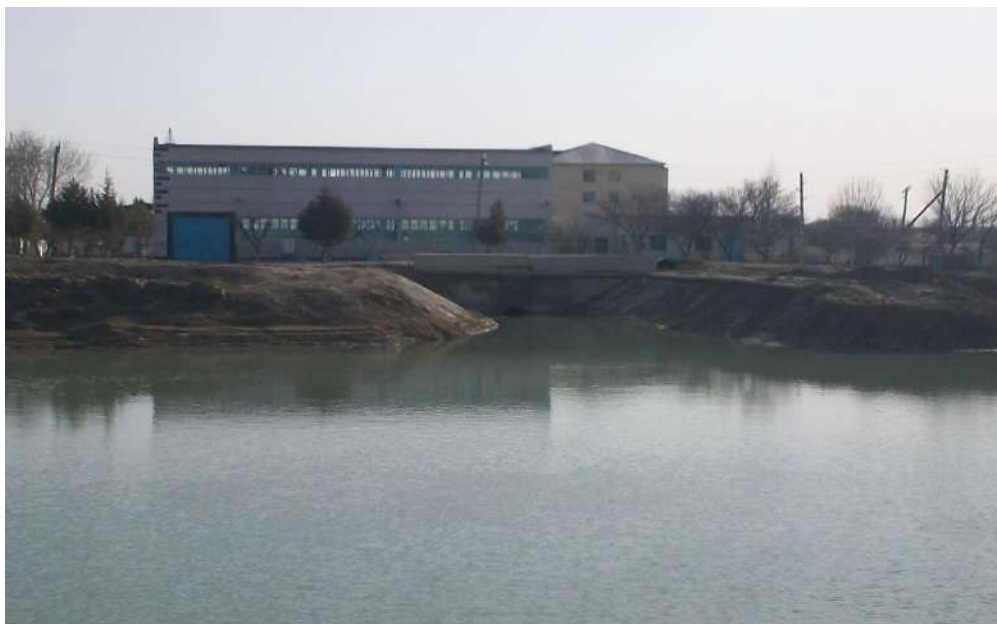
Figure 1.2 water intake point from the main channel against the satellite pumping station
