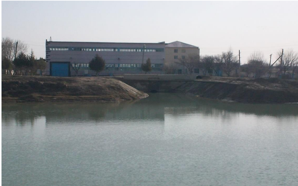
Figure 1.2 water intake point from the main channel against the satellite pumping station
