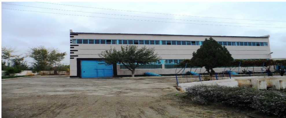
Figure 1.1. Main building of the pumping station” satellite
