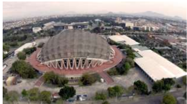
Figure 4. Sports Palace in Mexico
