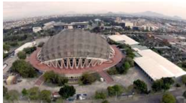
Figure 4. Sports Palace in Mexico
